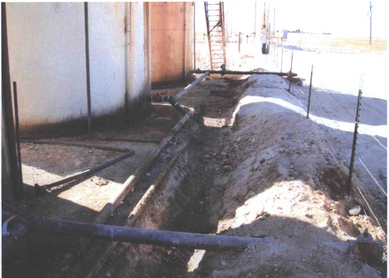
COG LOWE 20 #1 TB 9/20/MTU - THE TB TRENCHING - IRP-4057
