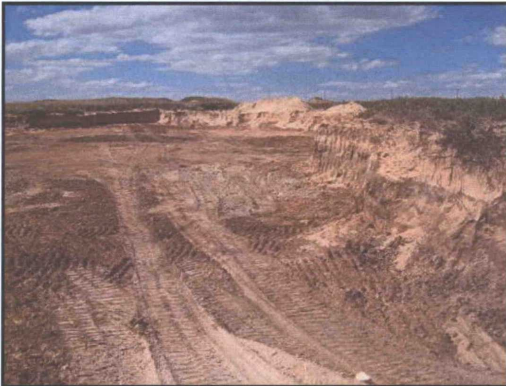
Test Trenches backfilled facing northwest
