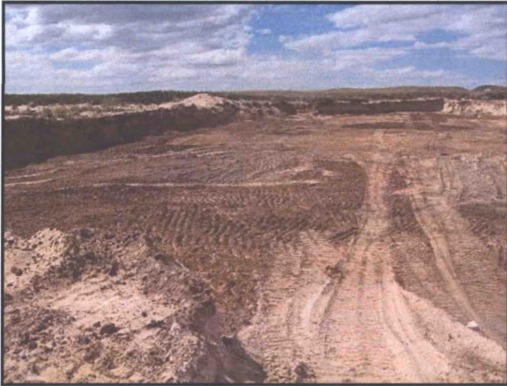
Test Trenches backfilled facing southwest
