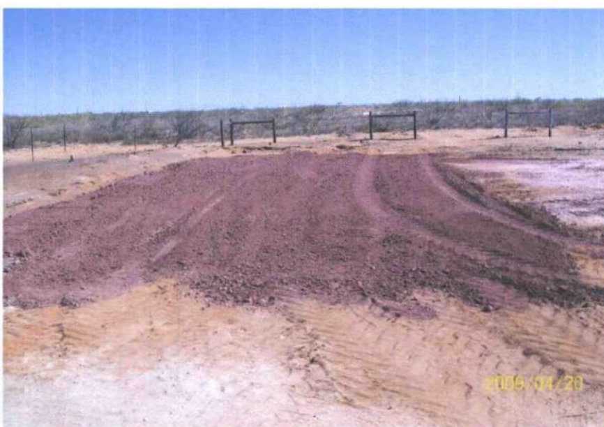
Compacted clay layer underlying new facility - approx 90 cu yds
