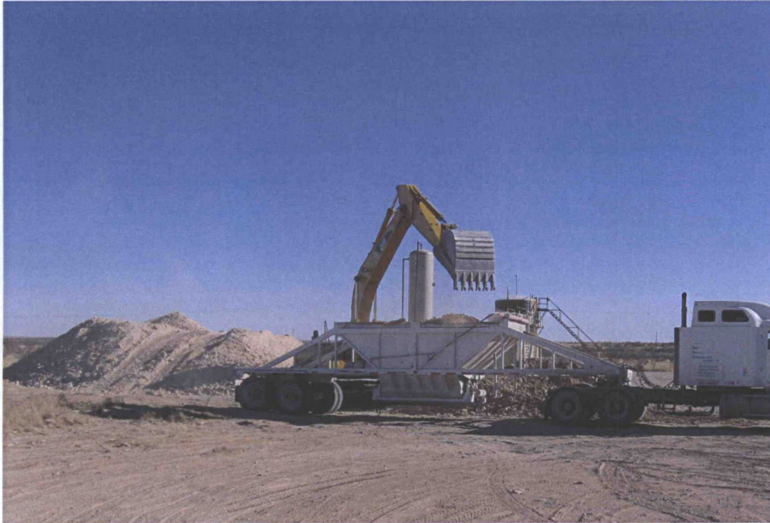
Photo No. 3: View to the northwest showing the chloride-contaminated soil being loaded for off-site disposal.
