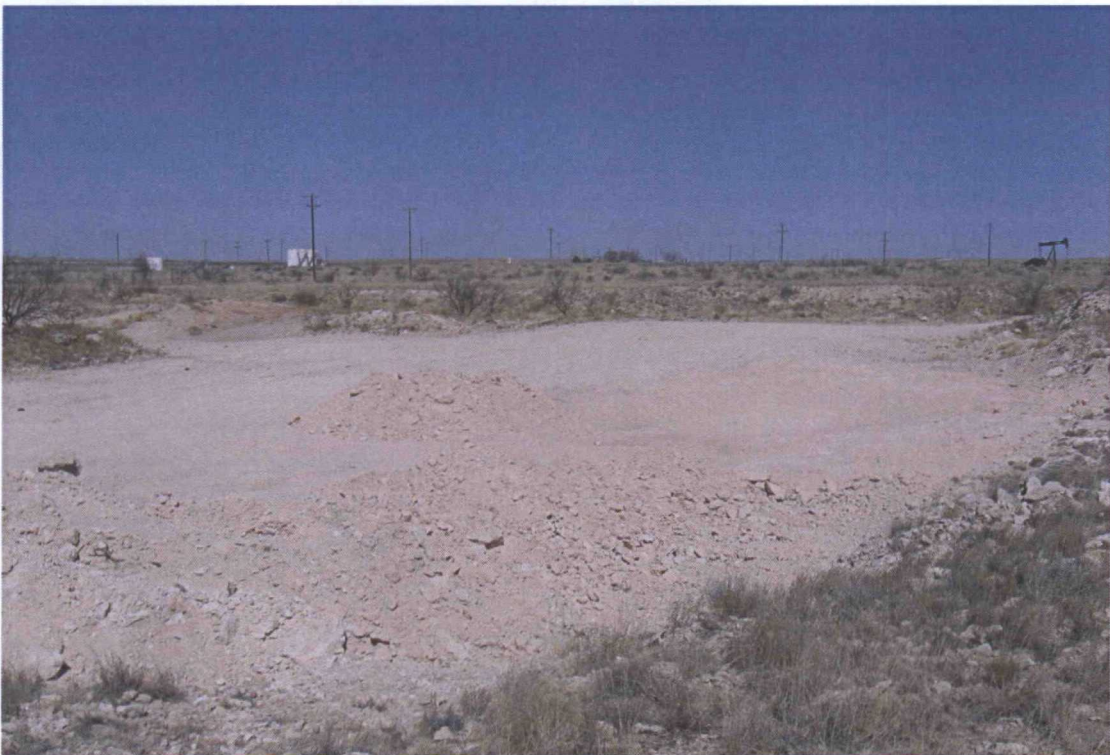
Photo No. 6: View to the southeast showing the excavation backfilled with caliche.
