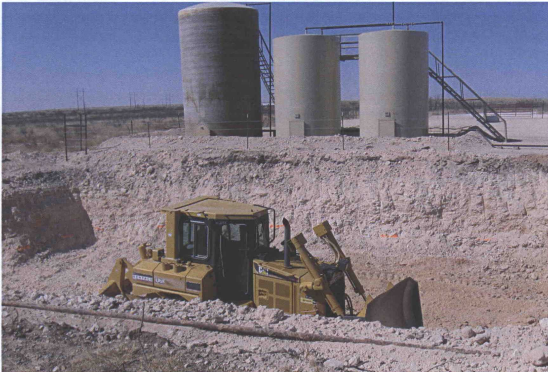
Photo No. 4: View to the west showing the excavation bottom being compacted by the dozer before placement of the clay liner. Note the orange clay liner fill marks on the excavation walls.
