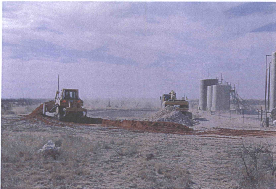
Photo No. 5: View to the south of red clay liner material being pushed into the excavation by the dozer.
