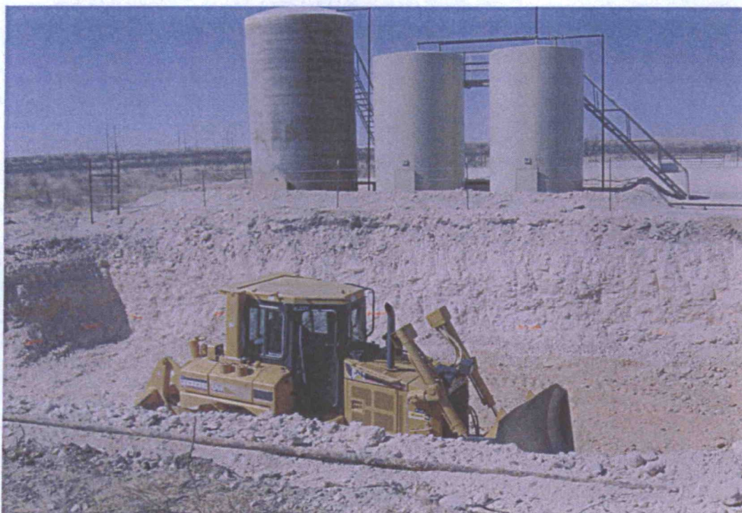
Photo No. 4: View to the west showing the excavation bottom being compacted by the dozer before placement of the clay liner. Note the orange clay liner fill marks on the excavation walls.
