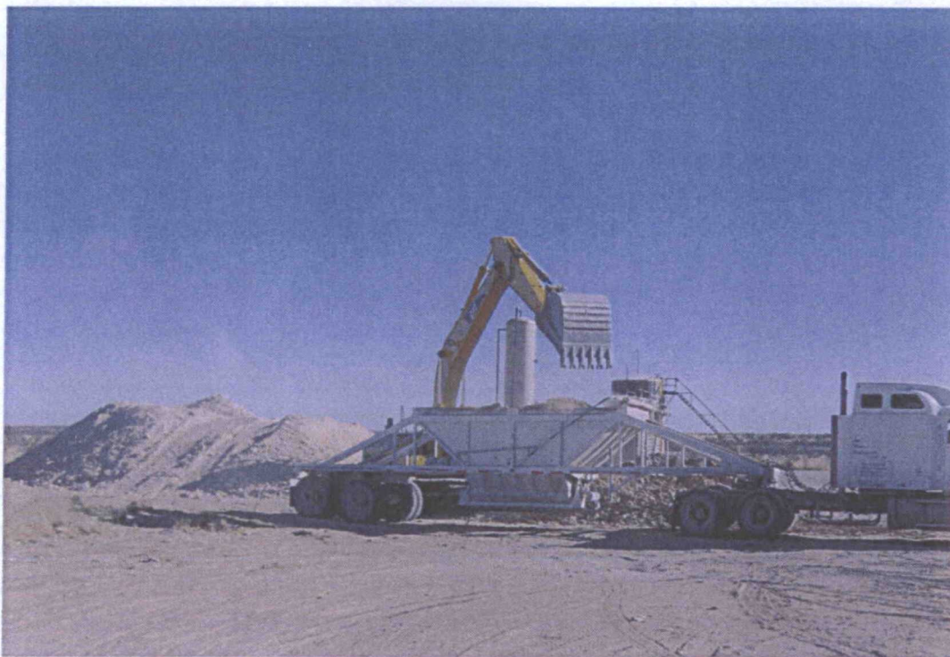
Photo No. 3: View to the northwest showing the chloride-contaminated soil being loaded for off-site disposal.
