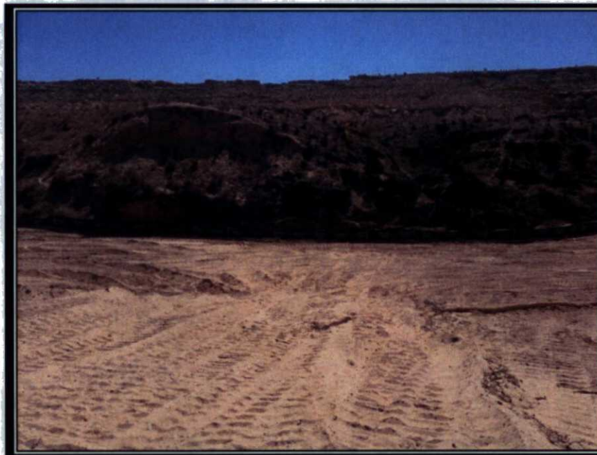
Photo 6: Excavated Soil from Arroyo View 1
