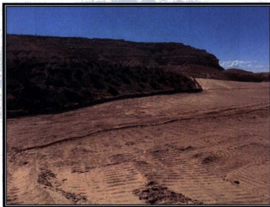
Photo 8: Excavated Soil from Arroyo View 3
