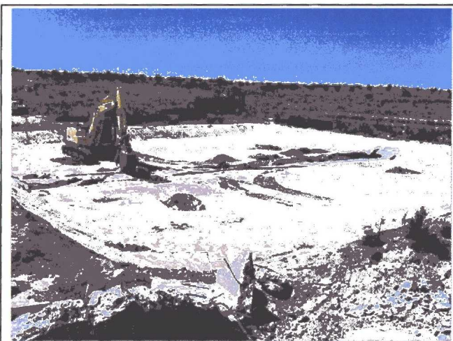
8.) General view of the soils underlying the bottom liner subsequent to the removal of all liners in the northern pond.
