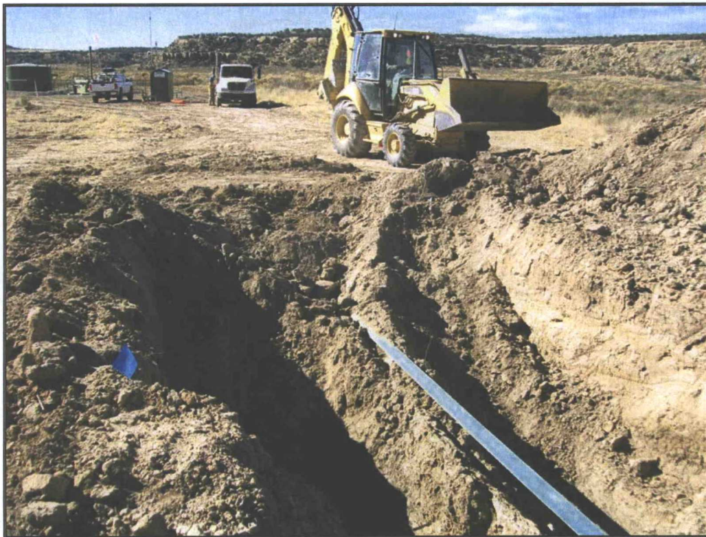
Photo 6: View of the excavation and loading of hydrocarbon impacted soils at the southern release.
