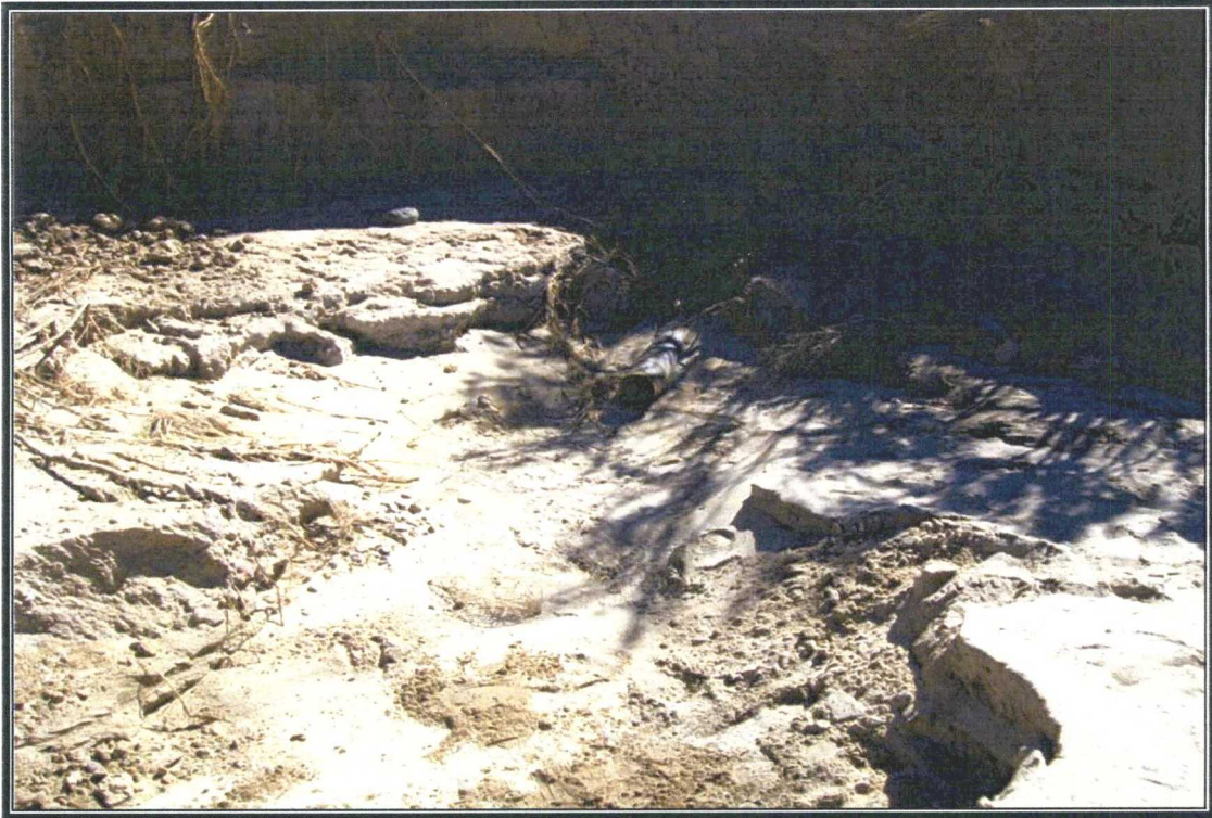
Photo 1: View of the severed pipeline and release area.
