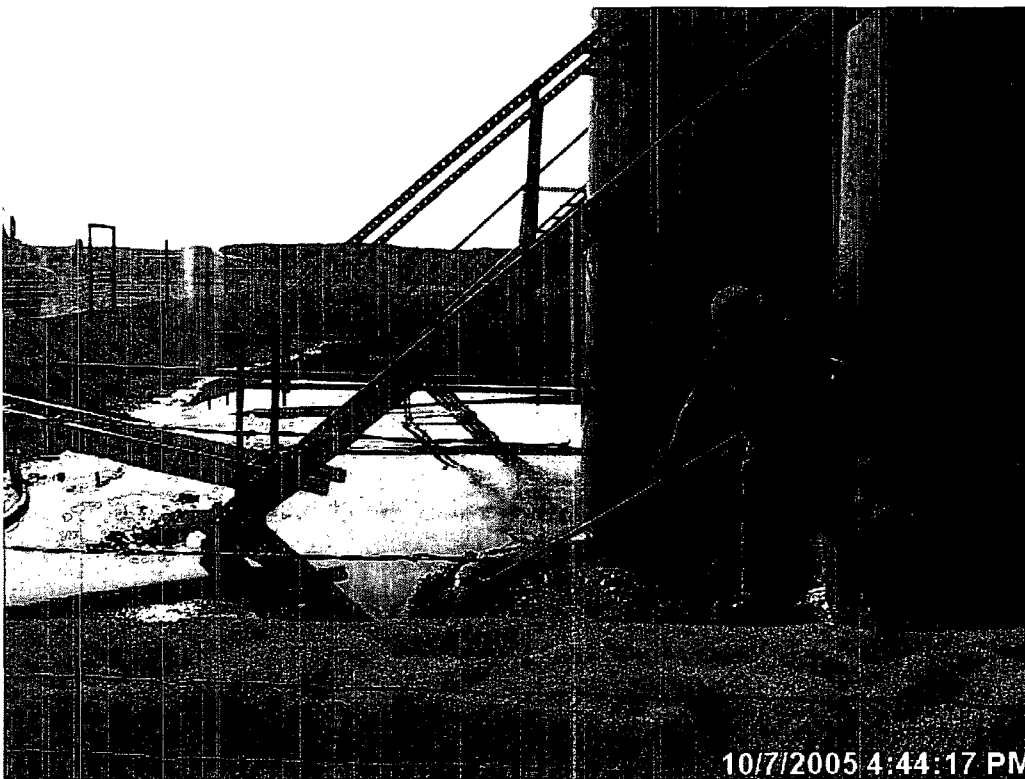
Photograph #4- Tank battery, fence, and berm looking westerly. Fluid and dark stained soil indicate contamination.
