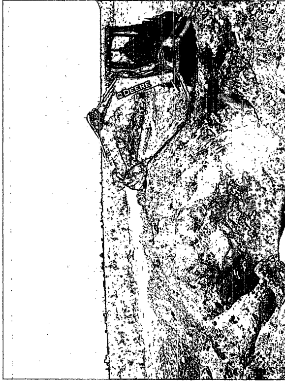
Excavating Clean to Blend with Contaminated Soil
