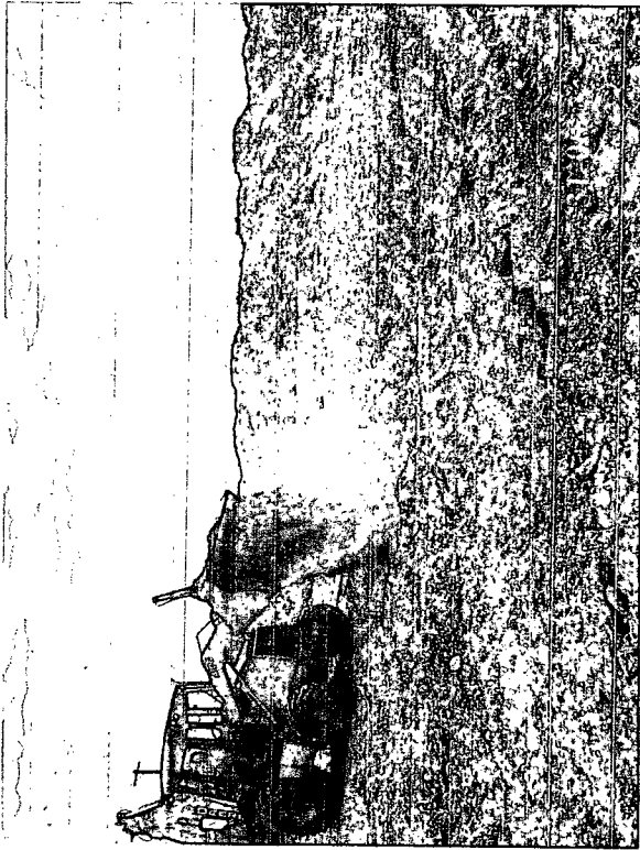
Backfilling Blended Material with Backhoe
