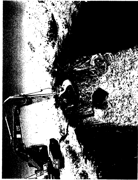
Placing solidified material in second burial pit.
