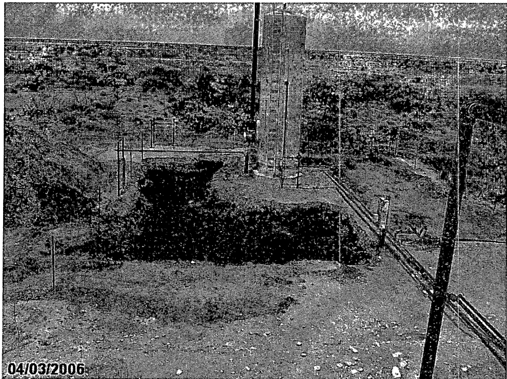
Photograph #4 – Looking northerly at excavation around heater treater.
