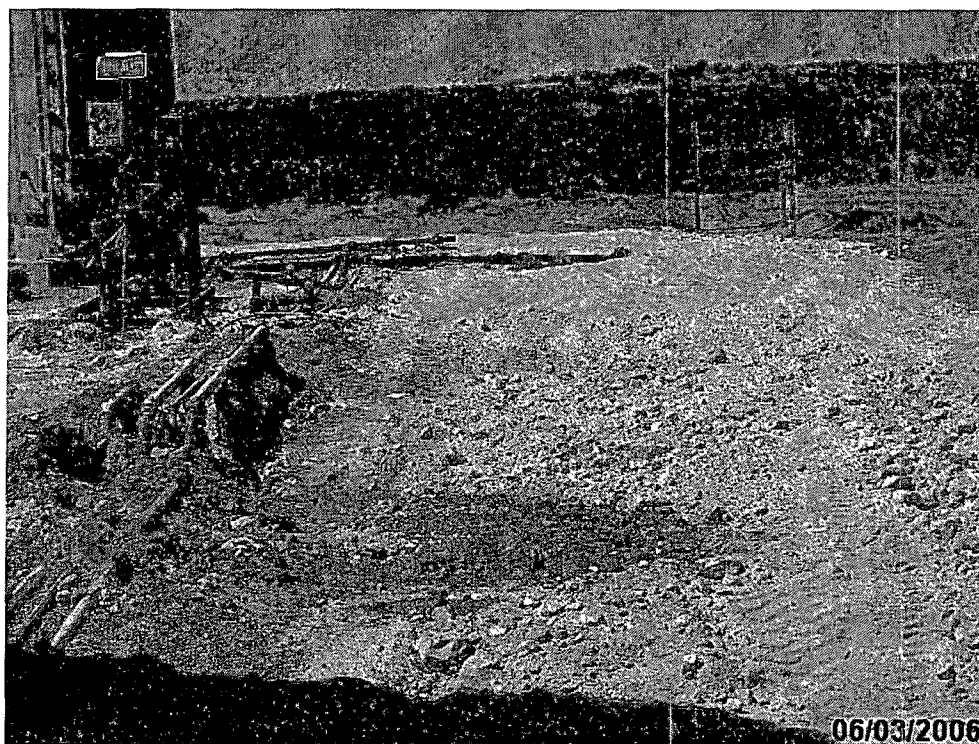
Photograph #8 – Backfilling excavation
