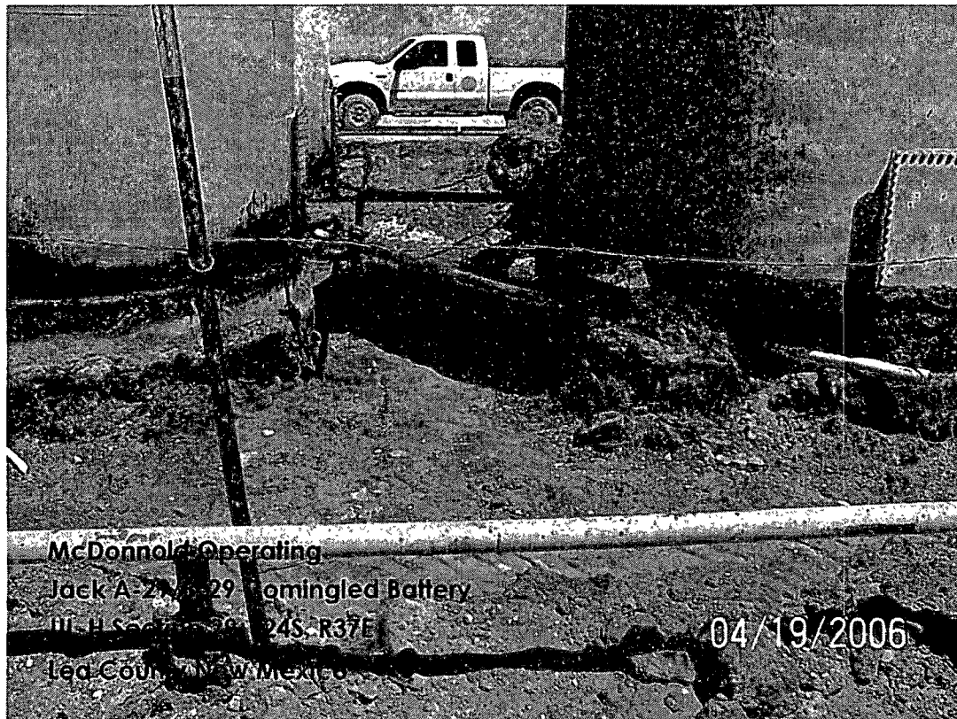
Photograph #3: Current excavation, looking north from south perimeter.
