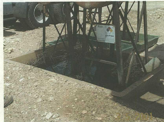
Pic # 12- Chemical storage tanks. Secondary containment has standing chemical and water.
