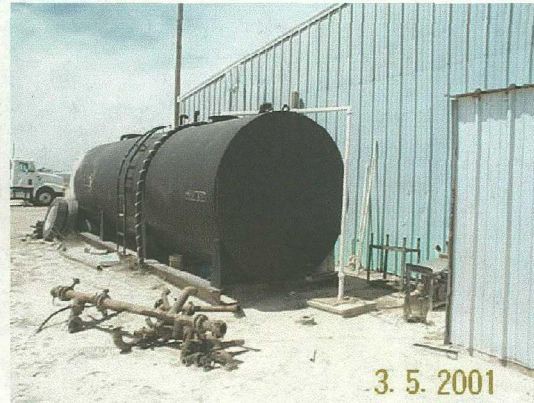
Pic # 5- Wastewater tank and sump receives water from washbay.
