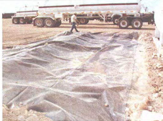
Image 4: Front of the used oil tank. Insufficient berms.
