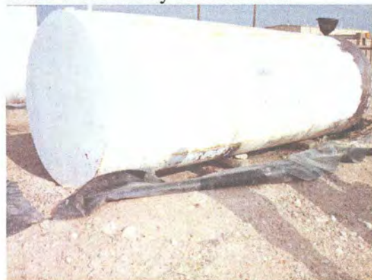
Image 2: Improper secondary containment lining under 'Used Oil' tank.
