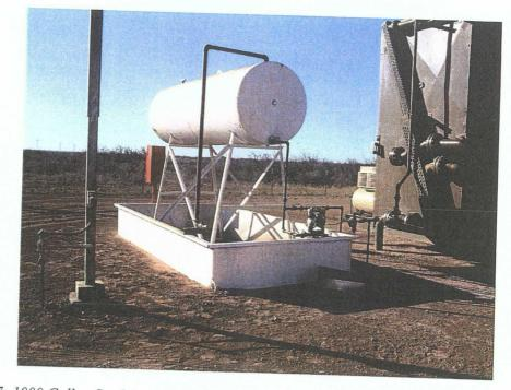
Figure 7: 1000 Gallon Steel Lubrication Oil Tank TK-5 and 1100 Gallon Steel Secondary Containment
