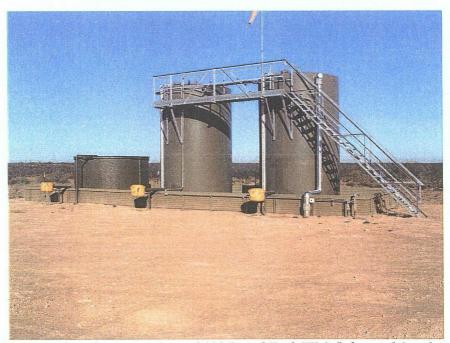
Figure 5: 210 Barrel Tanks TK-1, TK-2 and 100 Barrel Tank TK-3 (left to right) and steel secondary containment structure.
