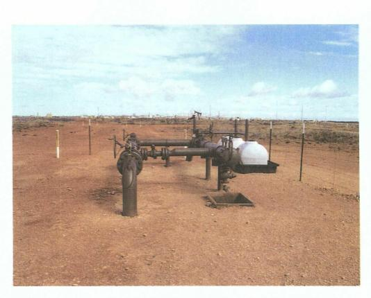
Figure 7: Pig Launcher and Fiberglass Drip Pan (Tanks TK-9, TK-10 and TK-11 in Background to Right)
