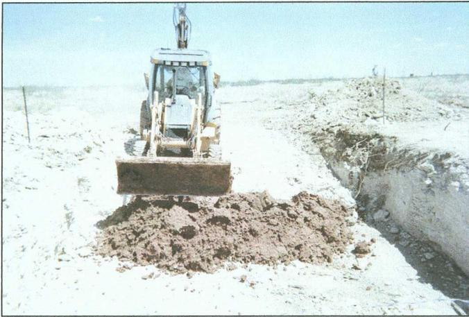
**Installing clay barrier at 6 ft: 4/13/2006**
