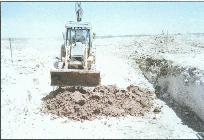
**Installing clay barrier at 6 ft: 4/13/2006**
