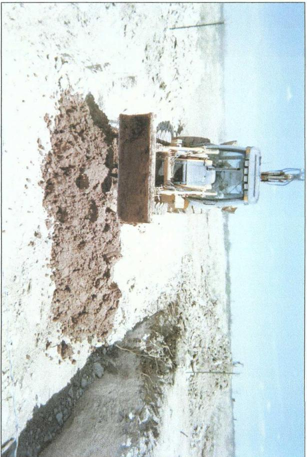
installing clay barrier at 6 ft
