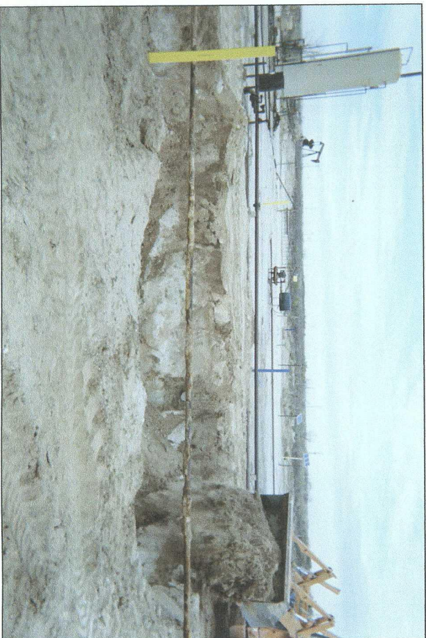
beginning backfill of 33 x 17 x 6 ft excavation
