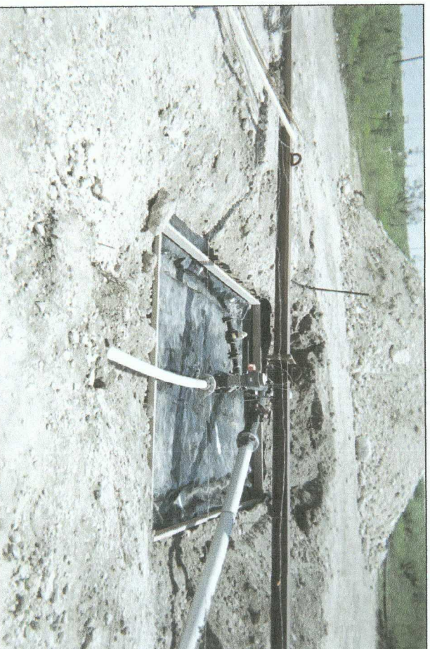
floor of new junction box with poly liner
