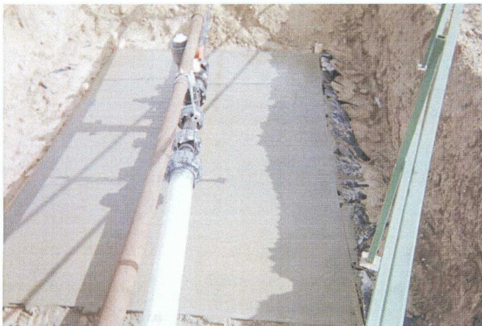
Photograph 2 – Floor of new concrete junction box.
