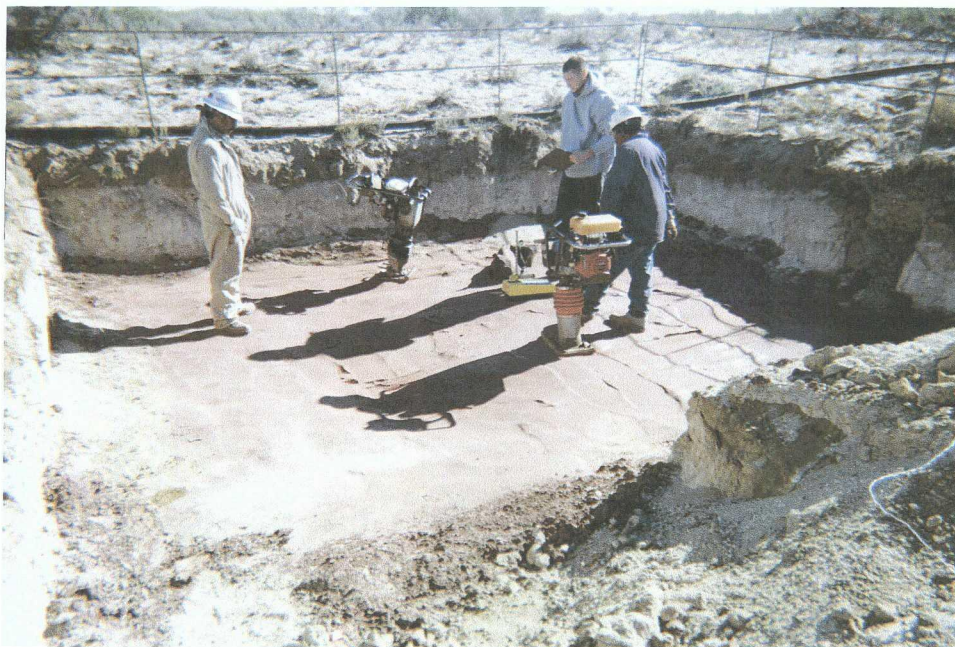
Figure 4 - Testing compacted clay: 11-20-2003.
