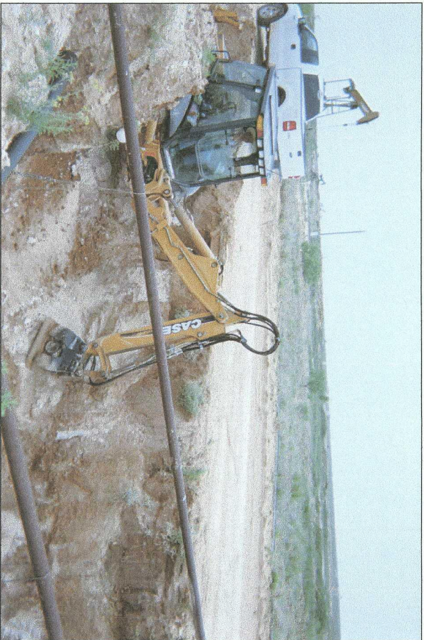
compacting backfill
