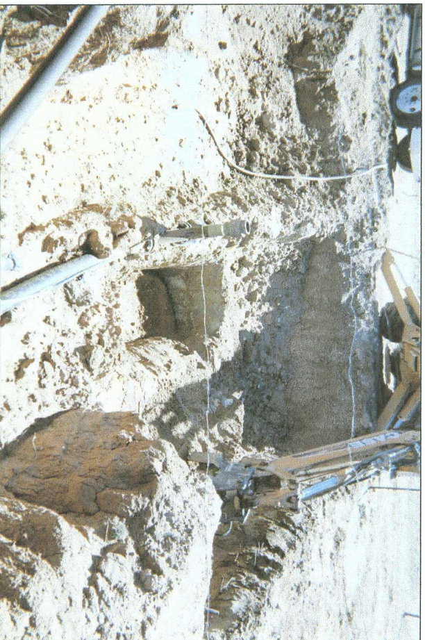
backfilling hole; preparing for new junction box
