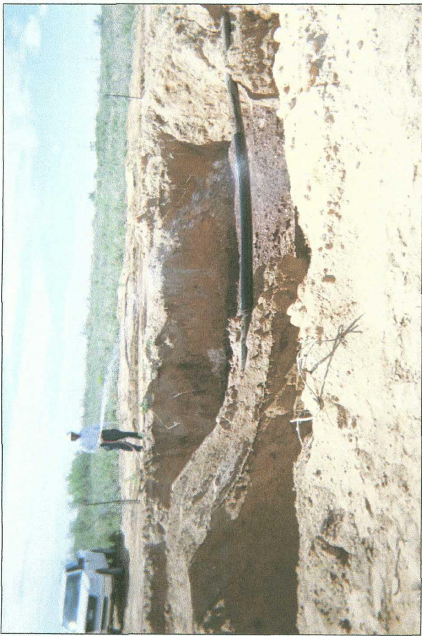
installing clay barrier at 6 ft BGS
