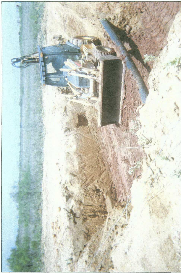
installing clay barrier at 6 ft BGS
