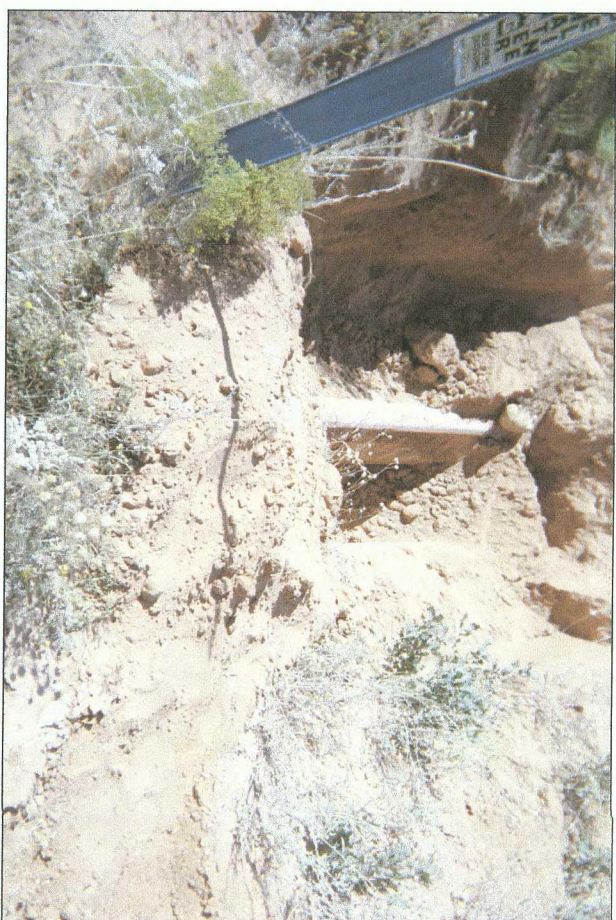
new plumbing; junction and box removed
