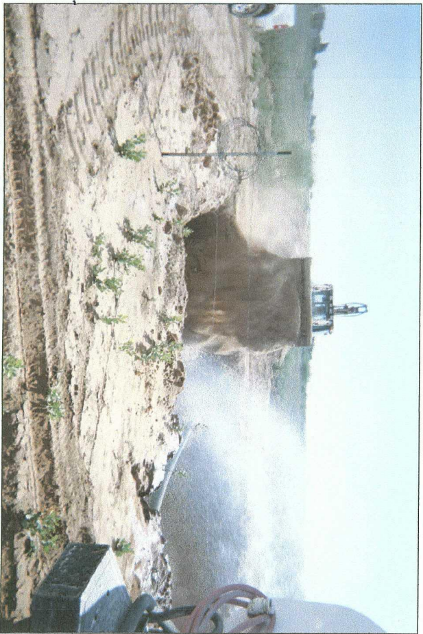
backfilling 30 x 25 x 12-ft-deep excavation Aug. 2006
