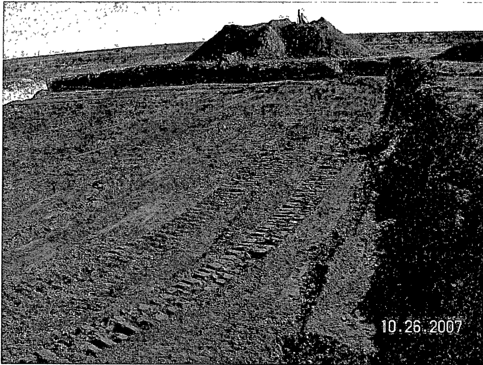
Photograph No. 4 – Looking easterly at backfilling of excavation area.
