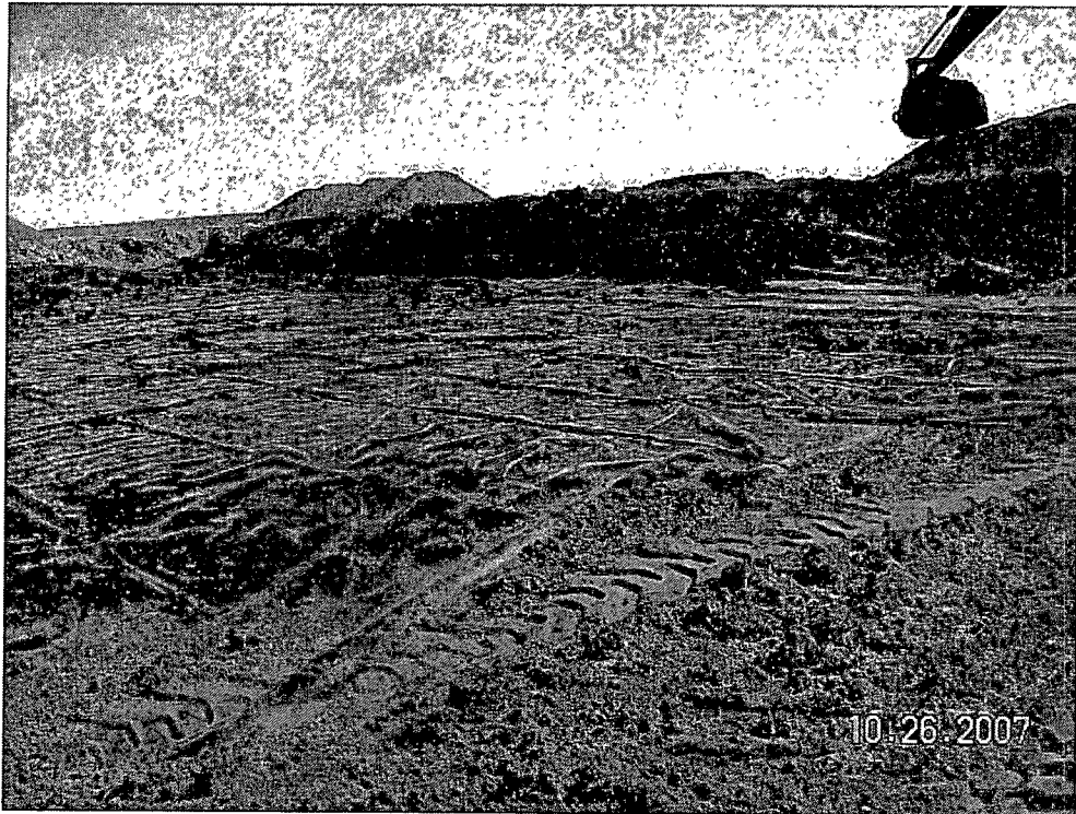
Photograph No. 8 – Looking northeasterly at liner and cushion material.
