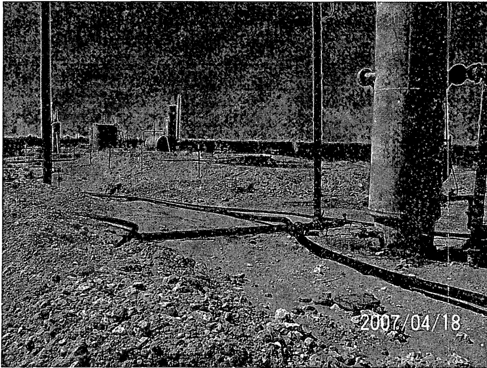
Photograph #4 – Bermed area around separator and decommissioned tank battery
