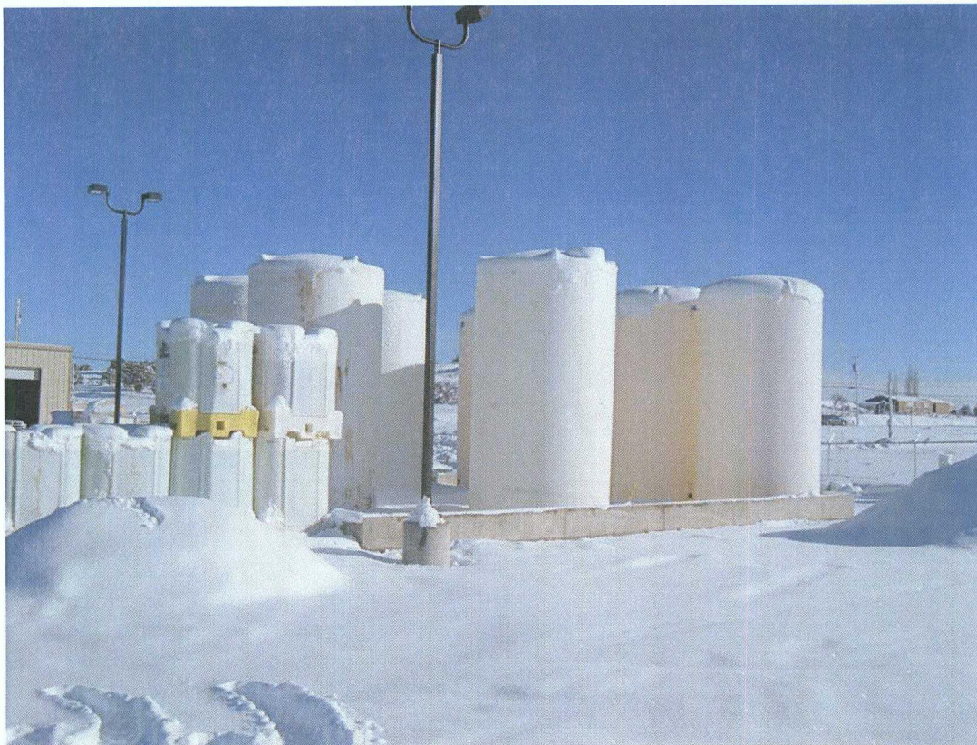
Figure 6: Photo: Bulk Tank Storage Area
