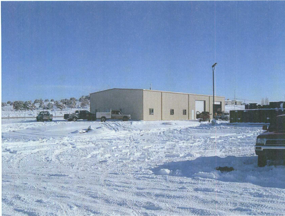
Figure 5: Photo: Aztec Warehouse and Drum Storage
