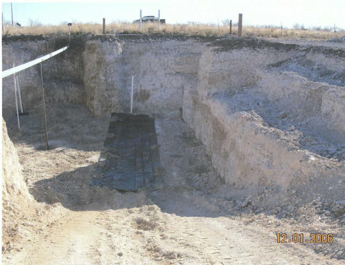
Photograph 5: Liner over south side trench.
