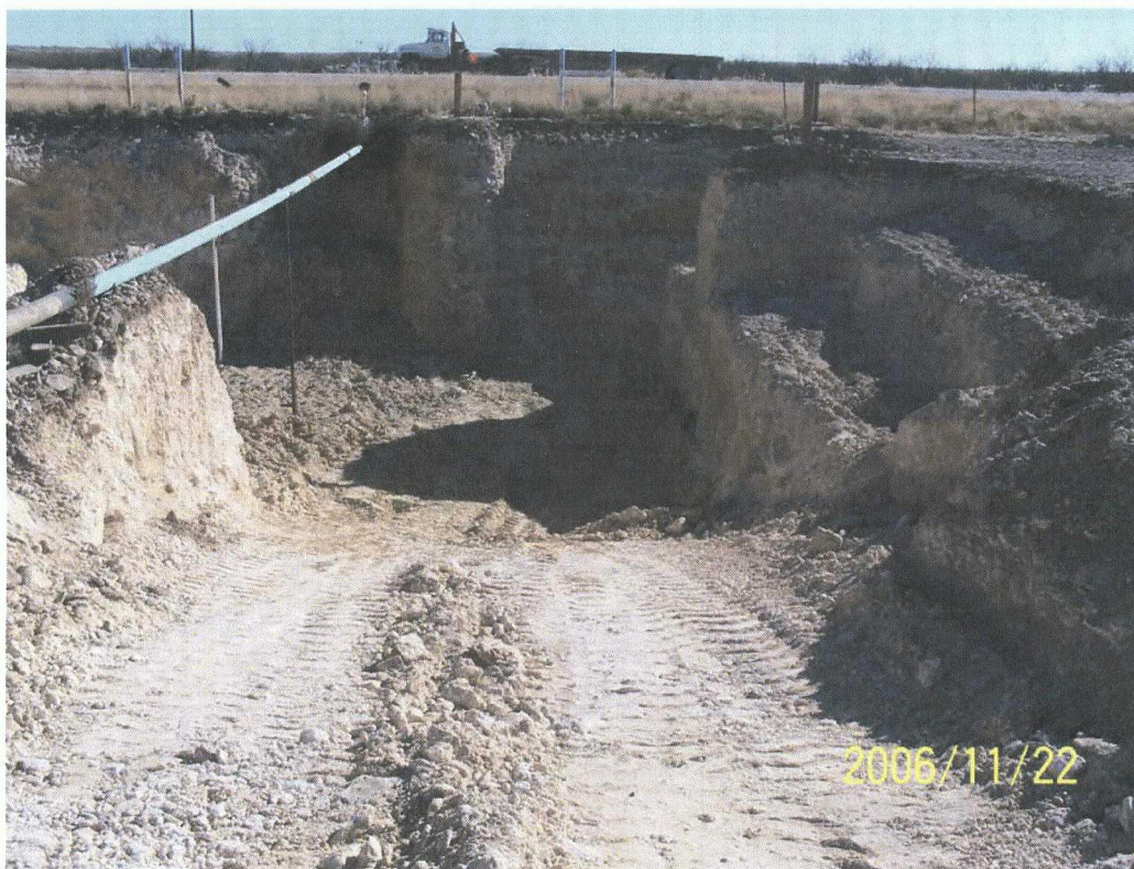
Photograph 1: Excavation of affected soil to 15 feet bgs.
