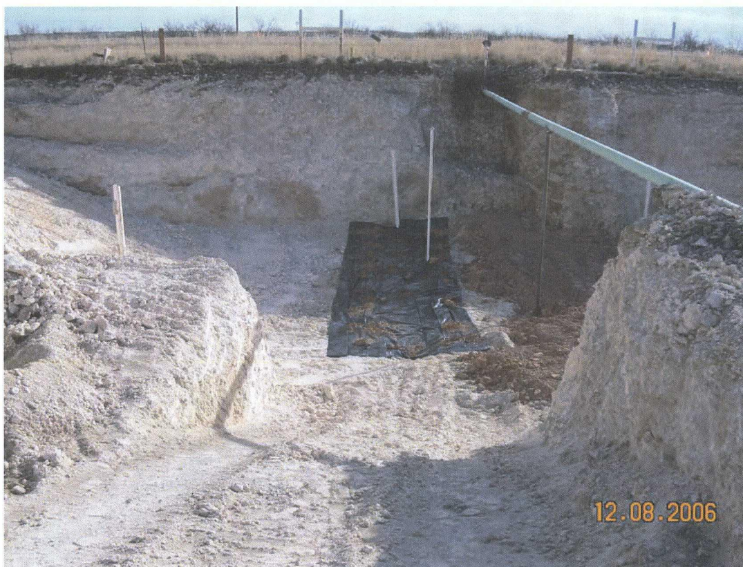
Photograph 4: Liner over north side trench.
