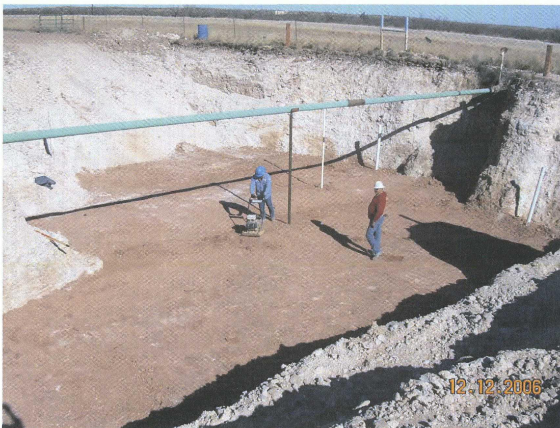
Photograph 6: Clay barrier installed at the base of the excavation.
