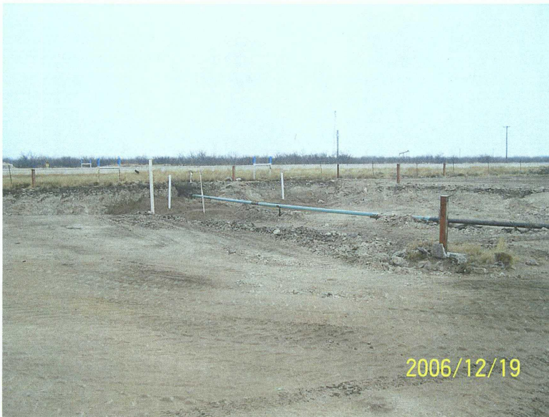
Photograph 7: Partially backfilled excavation with PVC risers for Passive Soil Vapor Ventilation System
