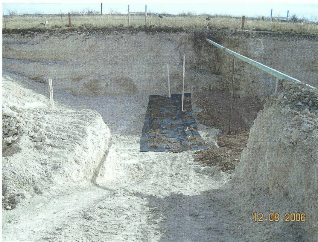
Photograph 4: Liner over north side trench.
