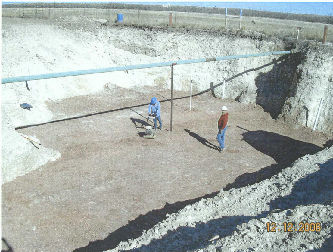
Photograph 6: Clay barrier installed at the base of the excavation.
