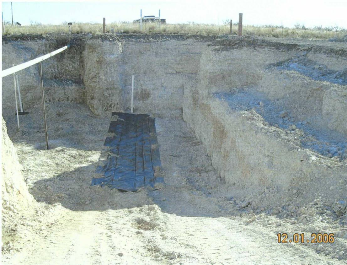
Photograph 5: Liner over south side trench.
