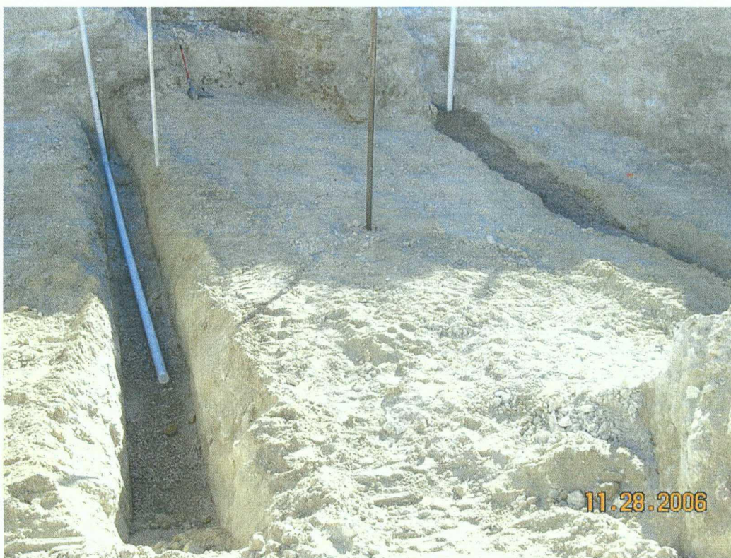
Photograph 2: Placement of horizontal slotted PVC pipe in trenches as part of the Passive Soil Vapor Ventilation System.
