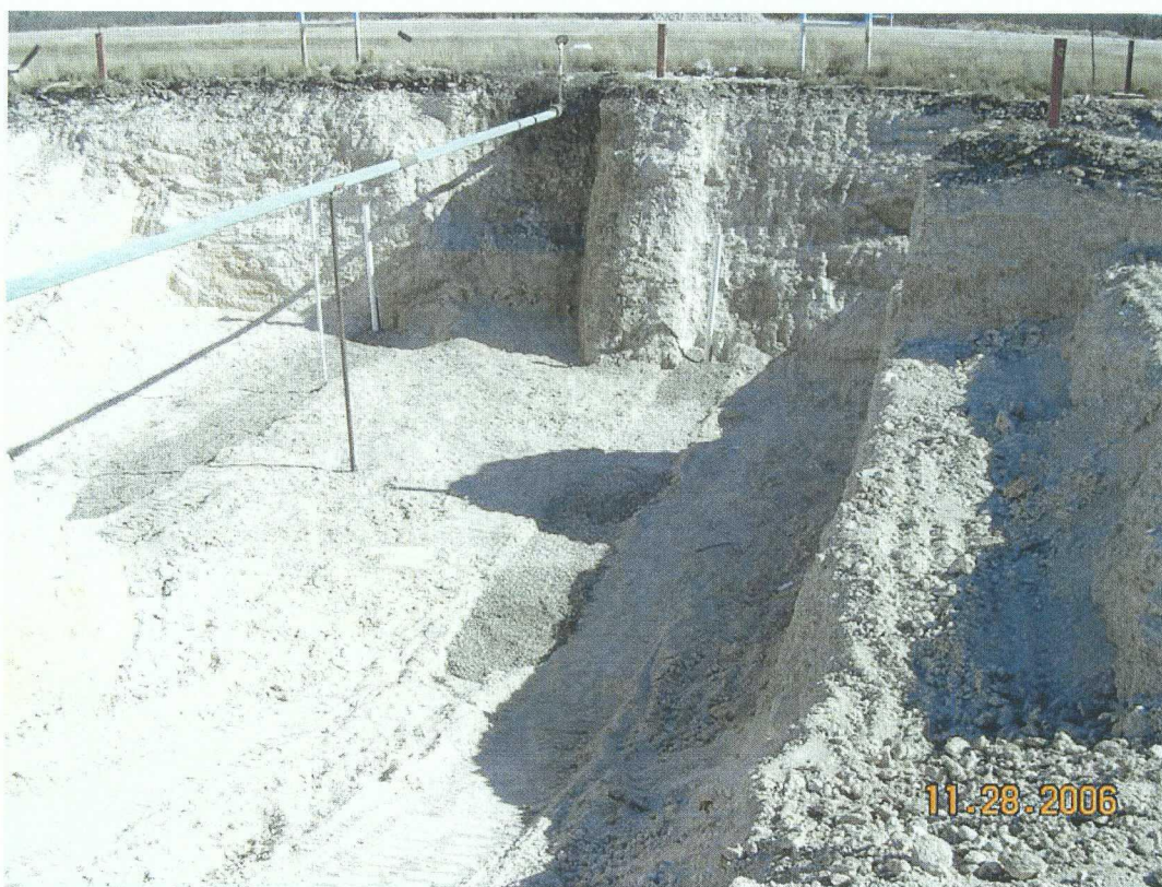
Photograph 3: 2'x2'x25' long trench with slotted PVC Pipe covered with coarse sand.
