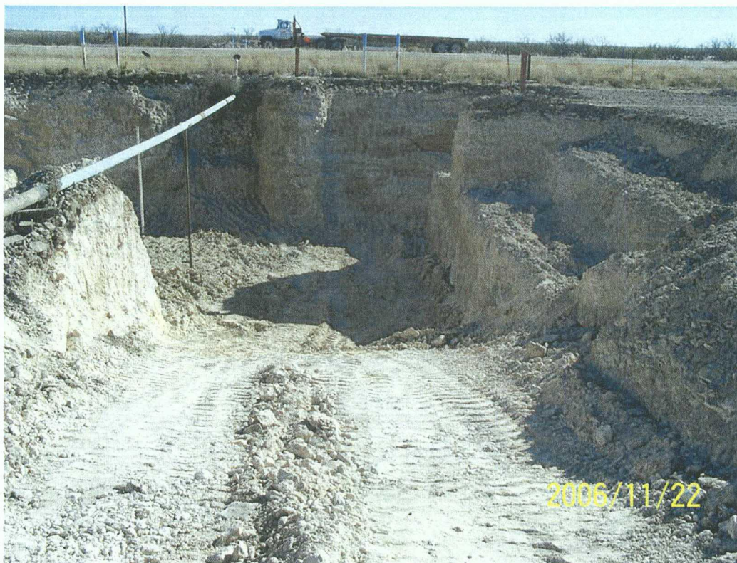
Photograph 1: Excavation of affected soil to 15 feet bgs.
