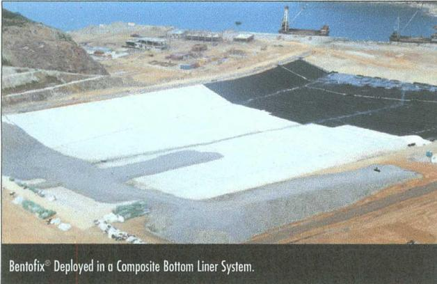
Bentofix® Deployed in a Composite Bottom Liner System.
