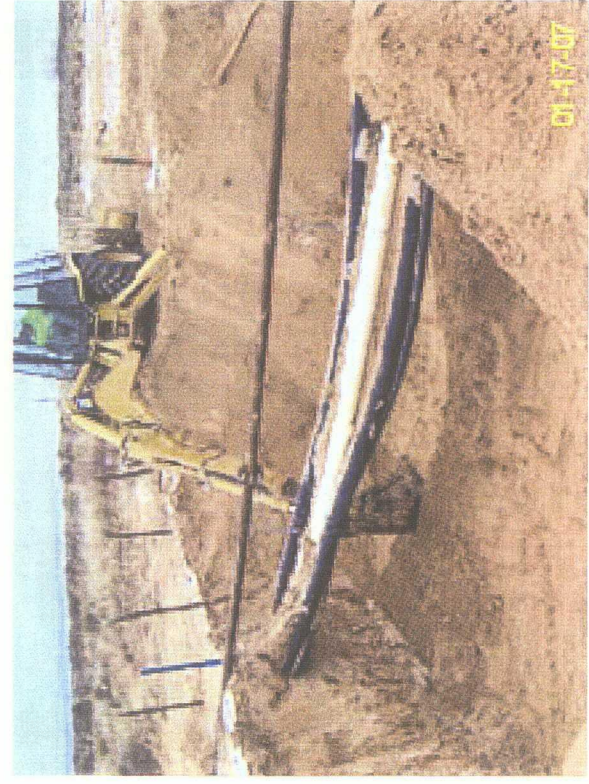
View facing south showing backfilling and tamping of blended soil on south side of excavation.
