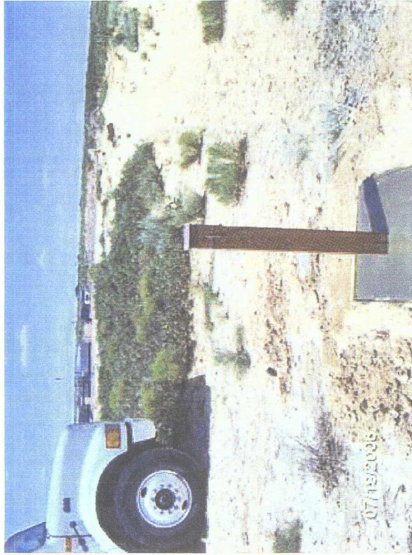
View facing north showing recently completed installation of downgradient monitoring well P6-3.
