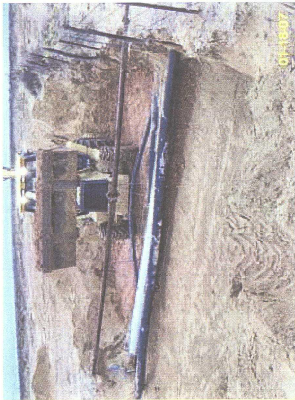
View facing north showing clay tamping activity on north side of excavation.
