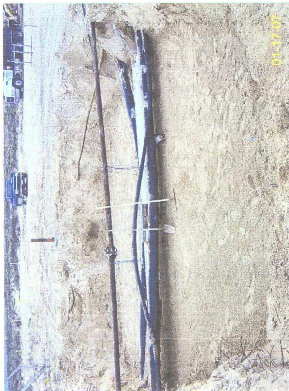
View facing south showing completion of lower backfill layer (blended soil) on south side of excavation.
