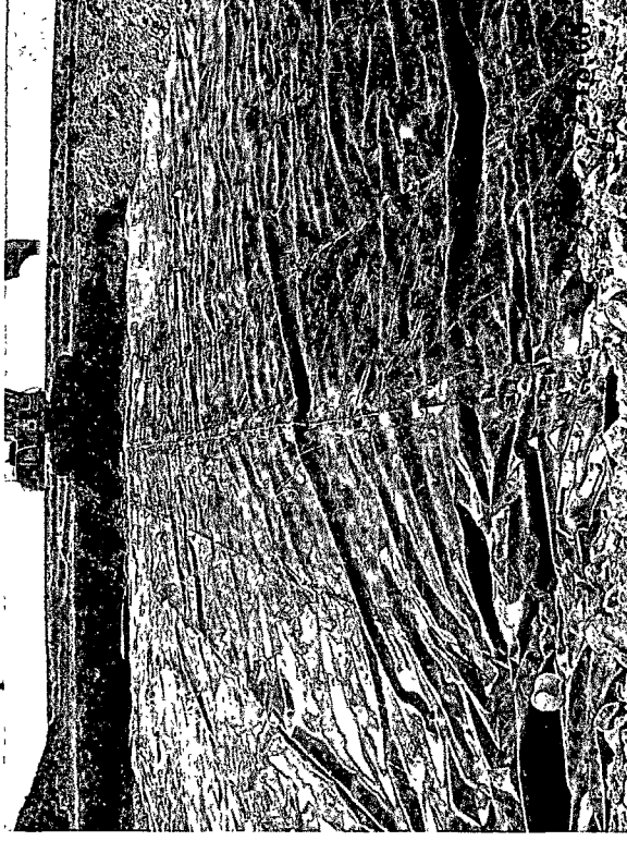
20 mil impervious liner installed at 6' below ground surface.
