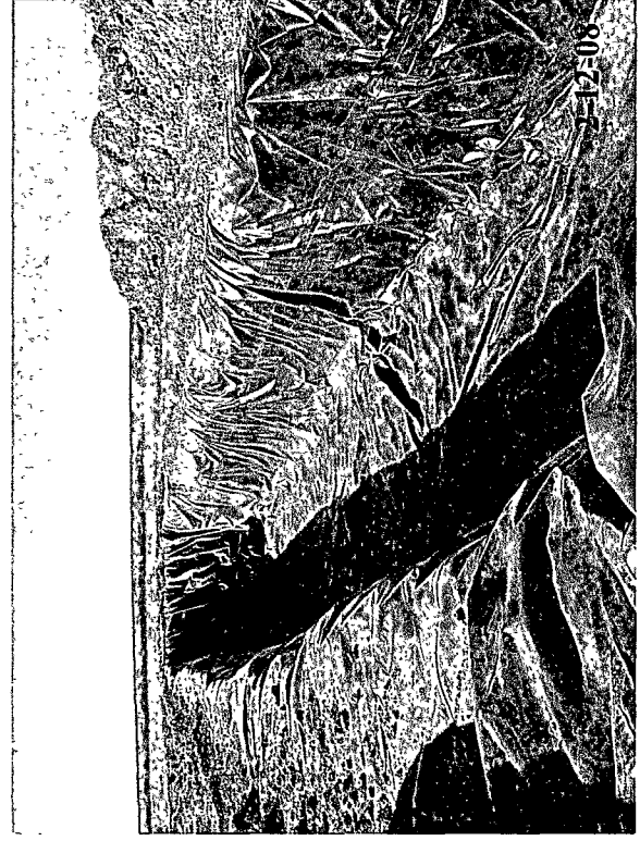
Burial pit after installation of 12 mil impervious liner.
