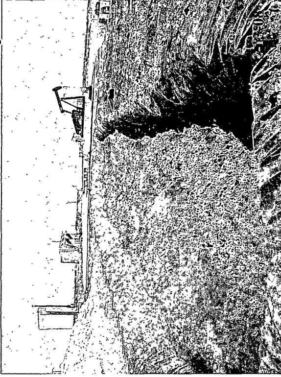
Burial pit full of drilling mud.
