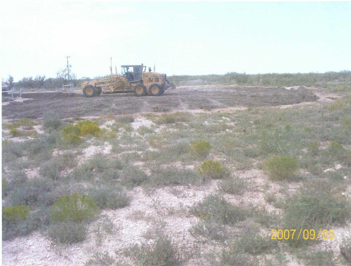
NORTH EXCAVATION: TOPSOIL BEING INSTALLED AND GRADED
