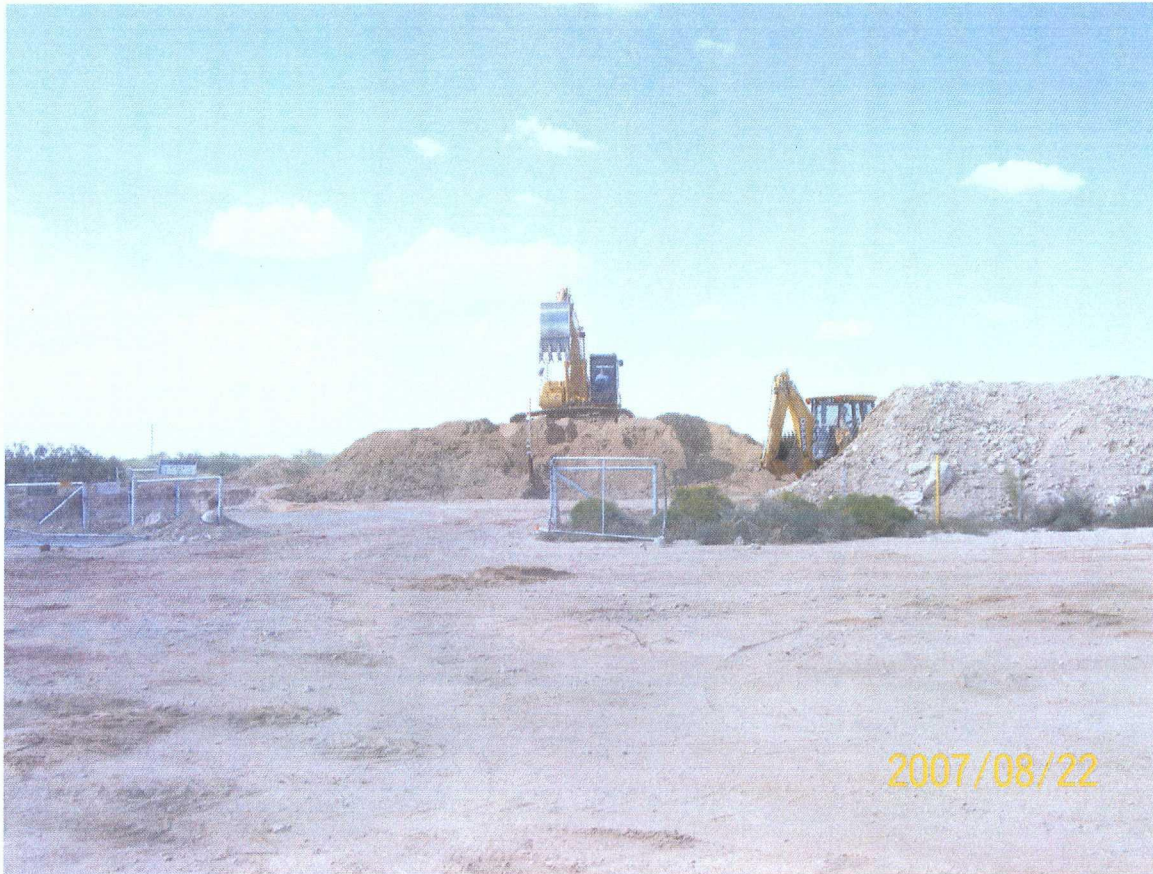
BLENDING THE BACKFILL
