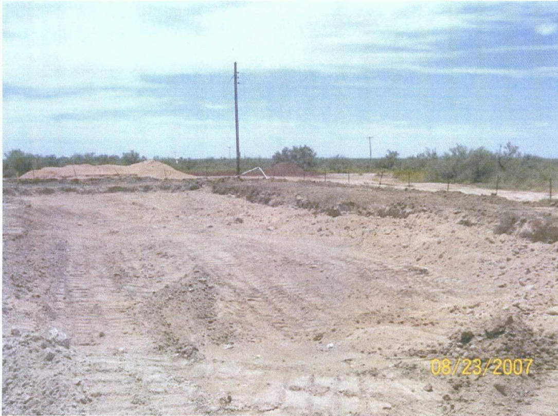
SOUTH EXCAVATION: 41 ft x 110 ft BACKFILLED TO 1 ft BELOW GRADE WITH BLENDED MATERIAL
