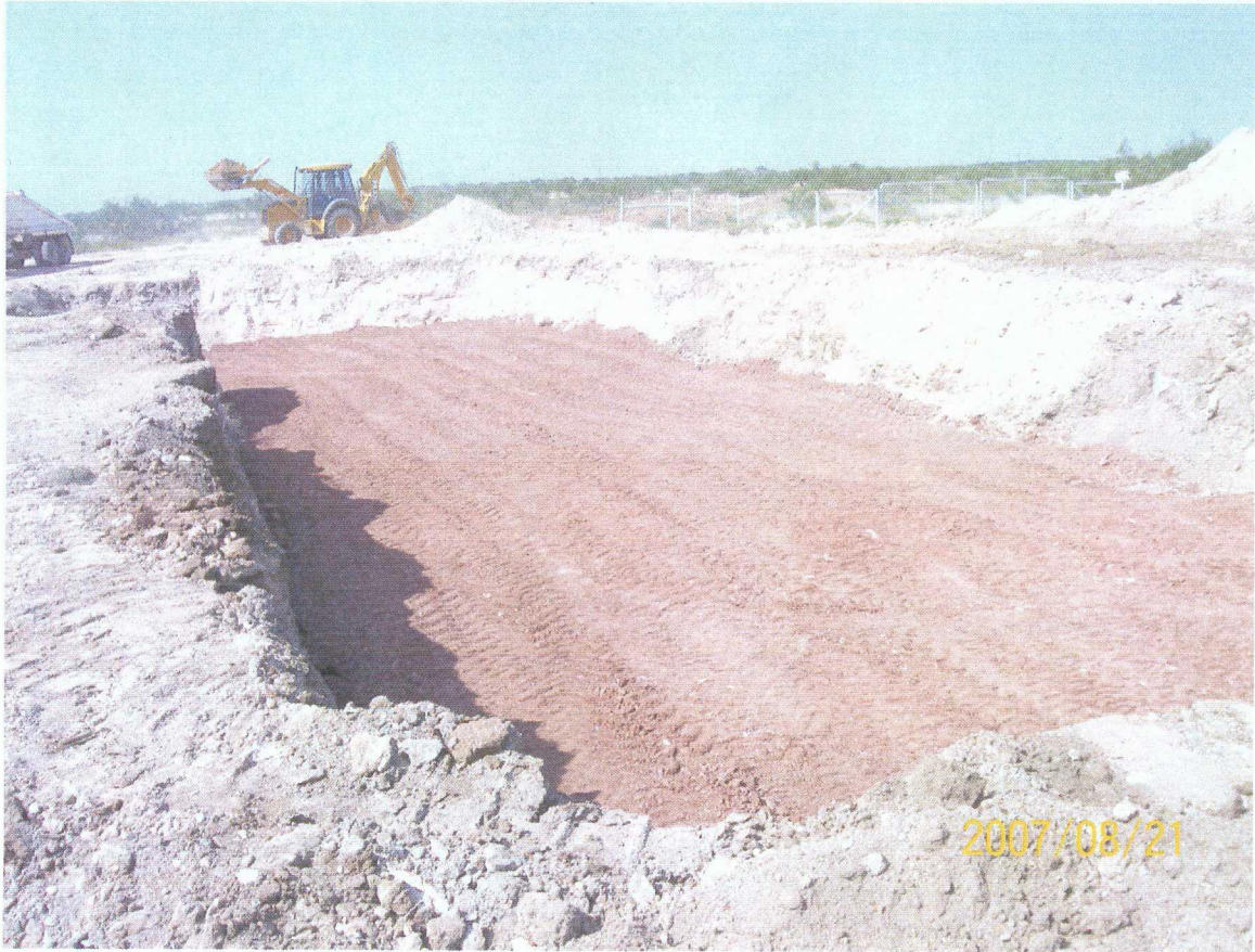
SOUTH EXCAVATION: CLAY LAYER AFTER INSTALLATION AND COMPACTION, INSTALLED @ 4-5 ft BELOW GROUND SURFACE
