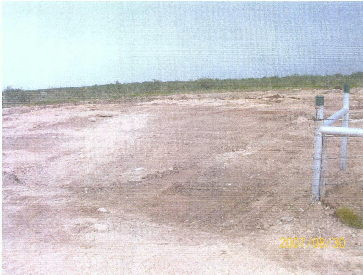
NORTH EXCAVATION: 142 ft x 85 ft BACKFILLED TO 1 ft BELOW GRADE WITH BLENDED BACKFILL
