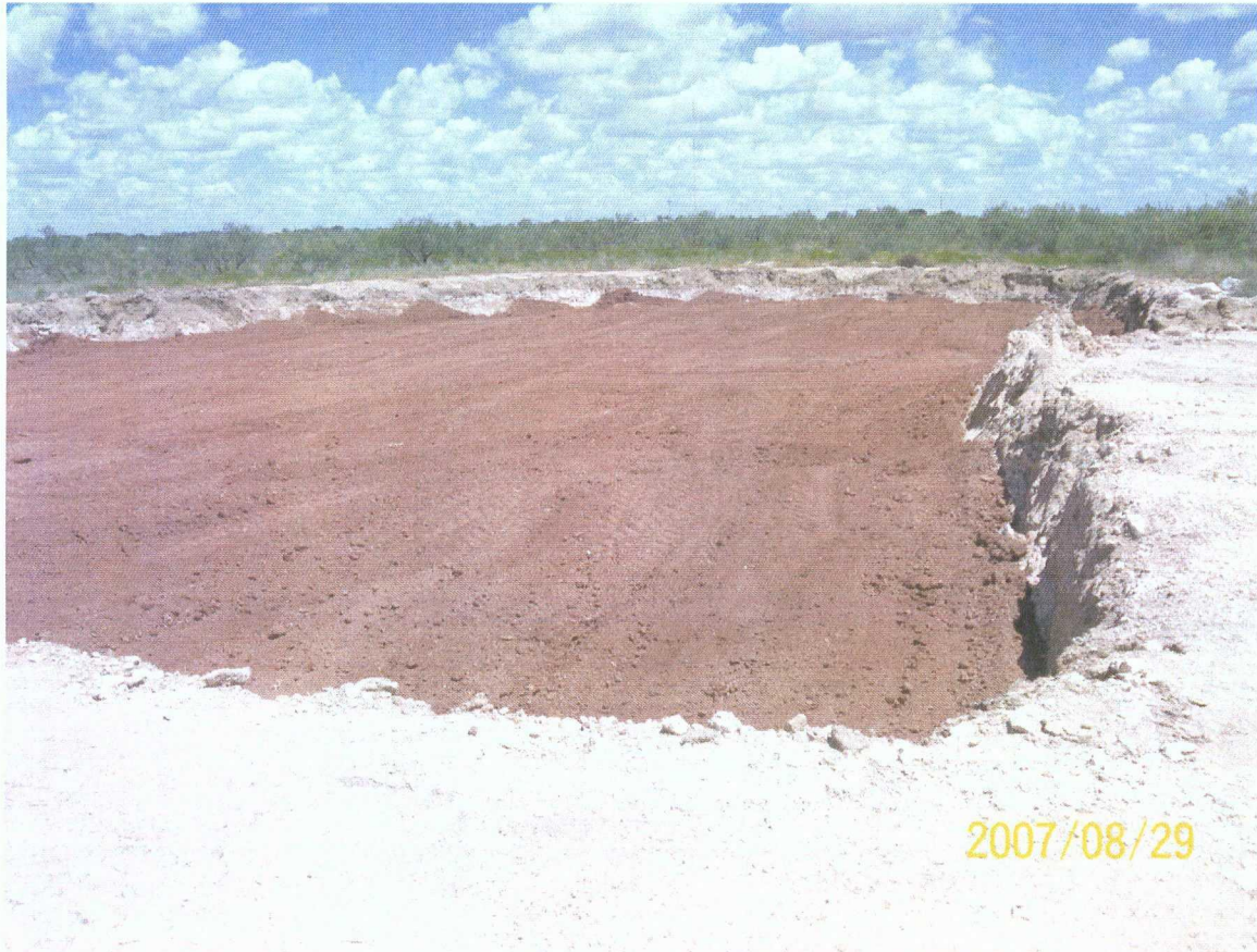
NORTH EXCAVATION: CLAY LAYER AFTER INSTALLATION AND COMPACTION, INSTALLED @ 4-5 ft BELOW GROUND SURFACE
