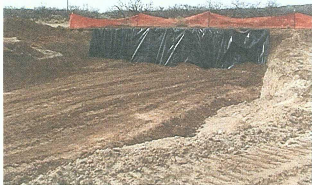
EAST SHELL NORTH - Backfill over liner
