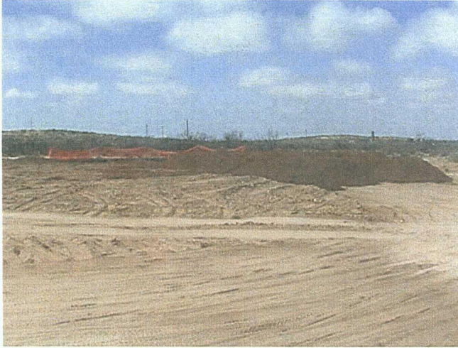
EAST SHELL NORTH - Final cover being placed over site
