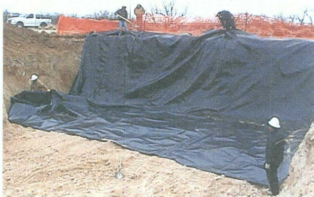
EAST SHELL NORTH - Liner placement
