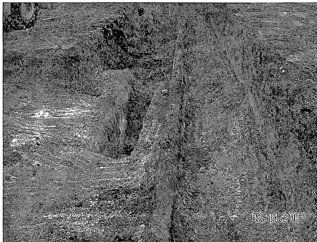
**Photograph #5:** Looking westerly at excavation and gas line. Dark stained soil indicates impacted soil.
