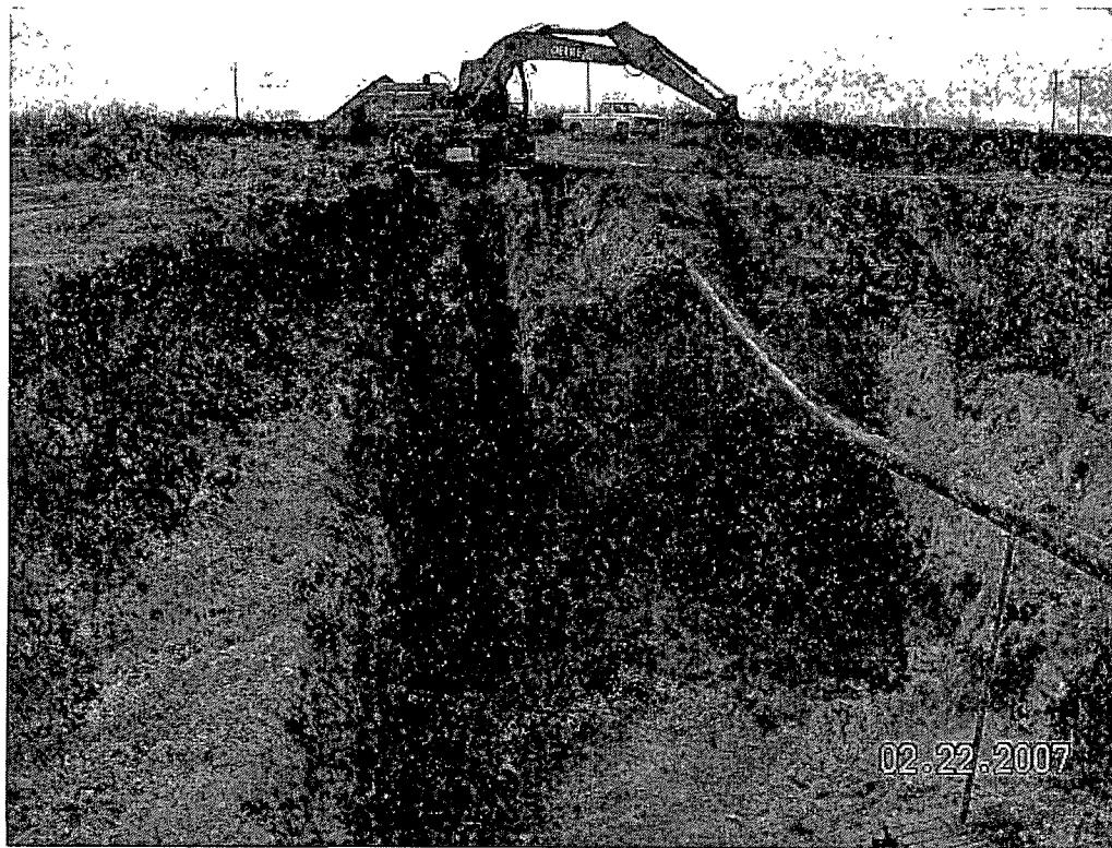
**Photograph #6:** Looking easterly at excavation and benching of sidewalls.
