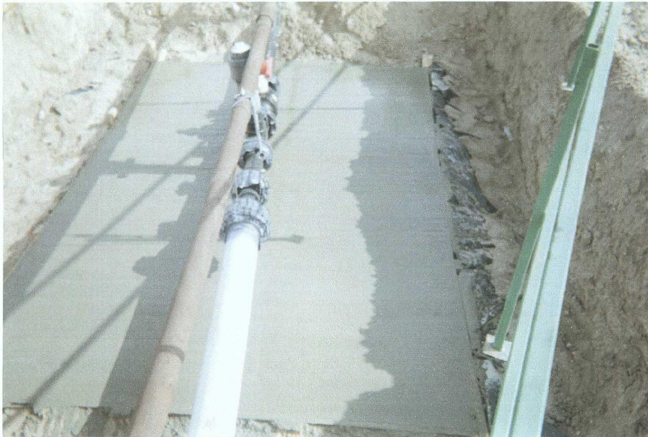
Photograph 2 – Floor of new concrete junction box.
