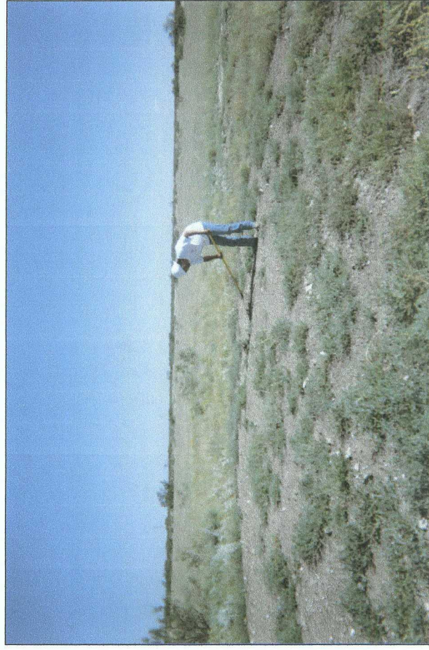
seeding disturbed area of backfilled site
