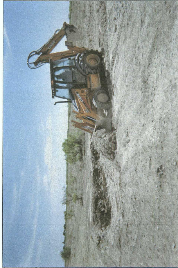
backfilling 20 x 15 x 12-ft excavation
