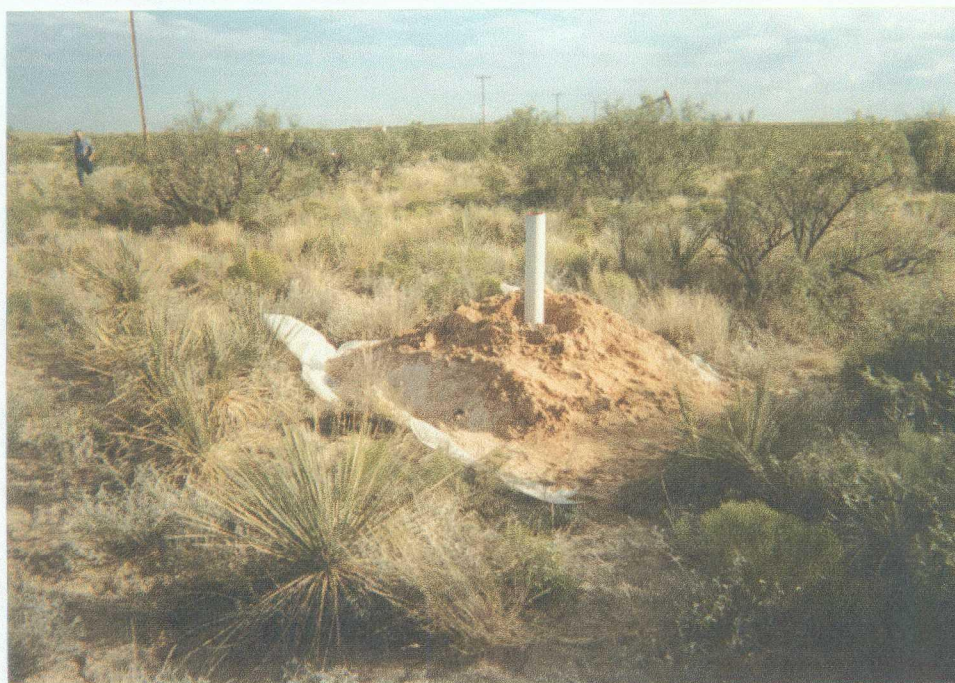
PHOTO 2: Monitoring Well Completion.
