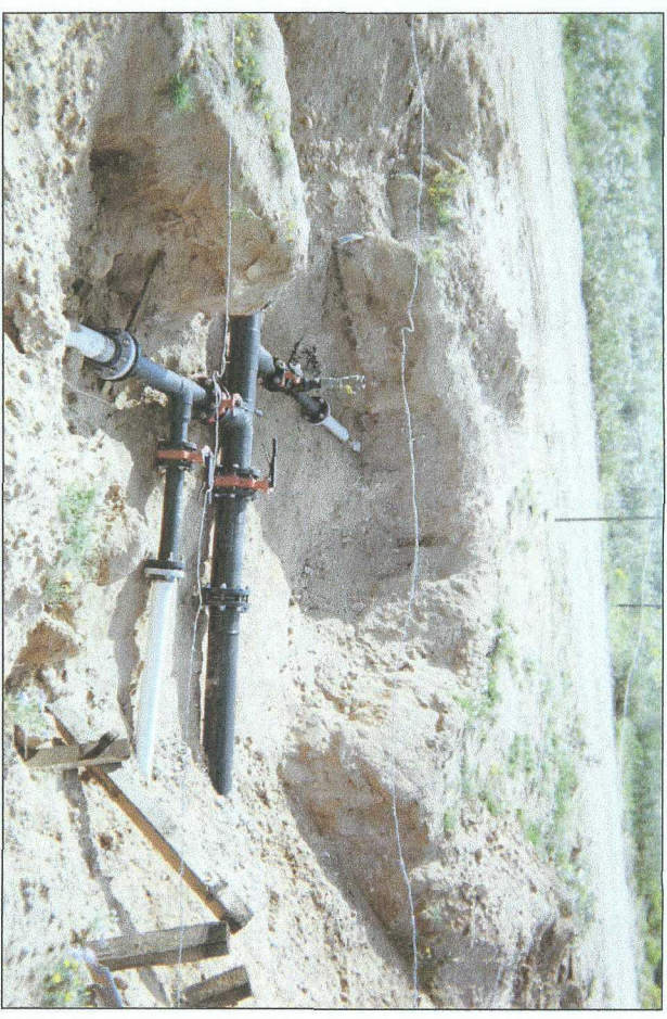
new pipeline and junction; old box removed
