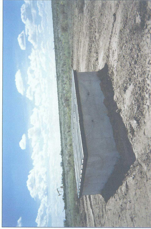
completed new junction box
