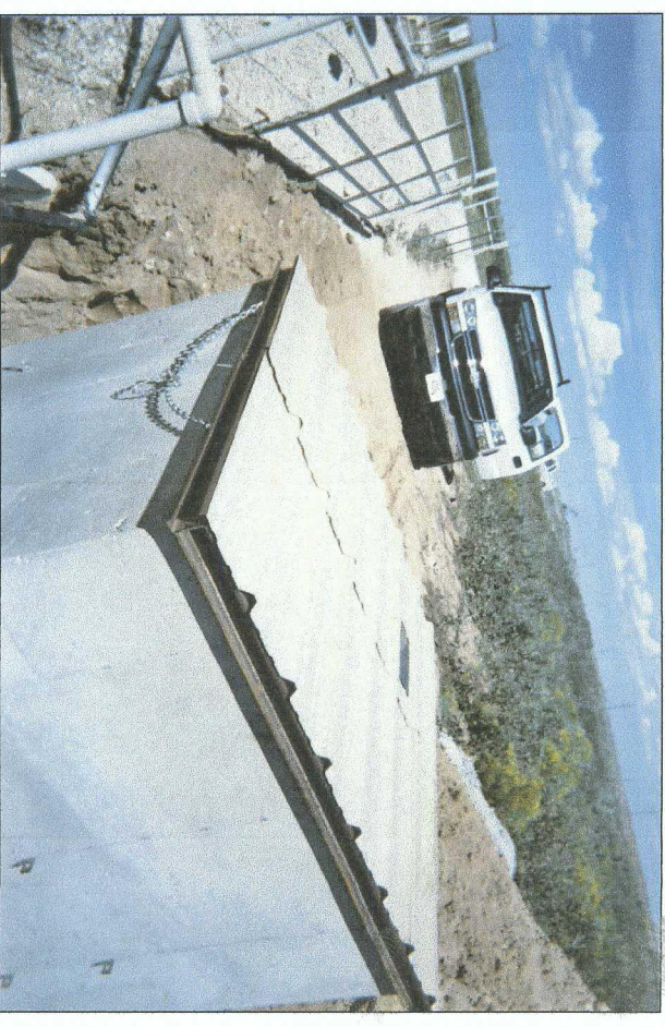
new concrete junction box completed in same location
