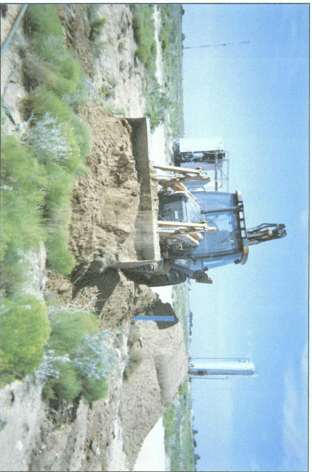
backfilling former junction site with clean, imported soil
