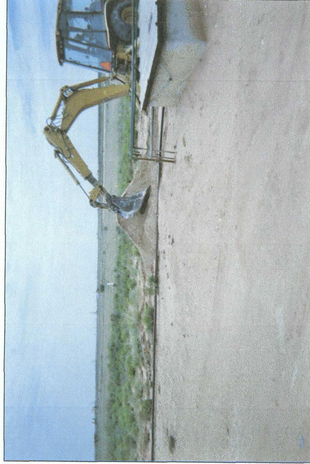
backfilling box hole with clean, imported soil
