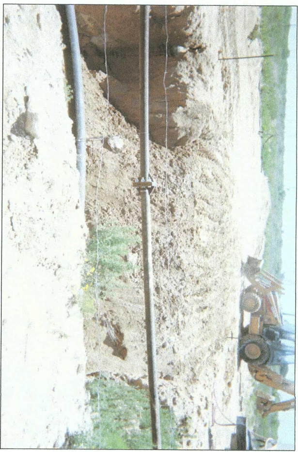
backfilling excavation
