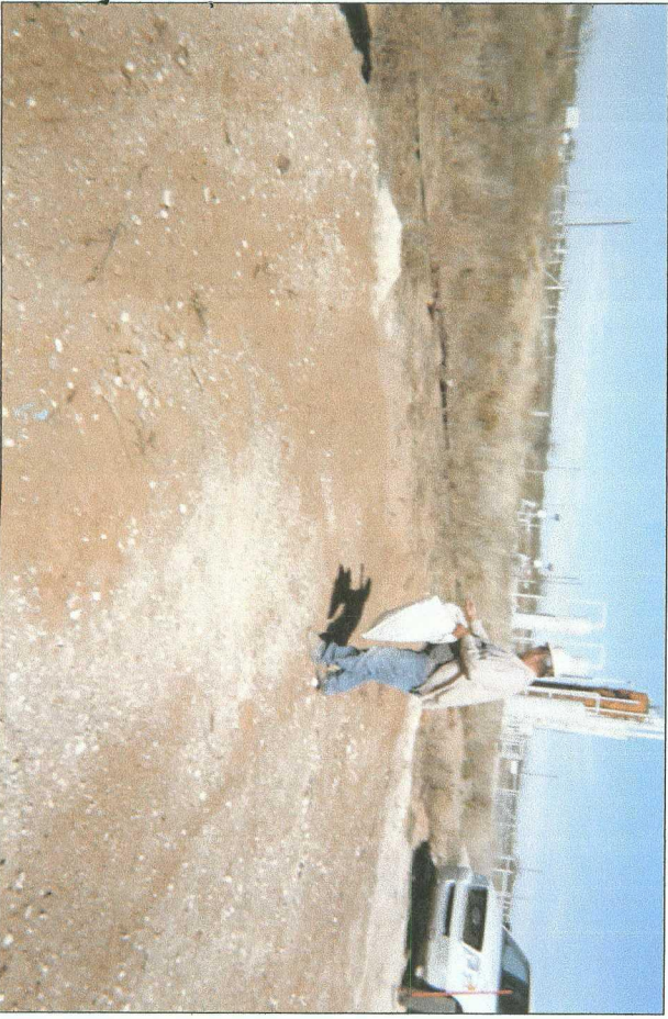
seeding disturbed surface of backfilled site
