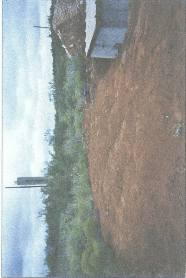
former junction box hole filled with clean, imported soil
