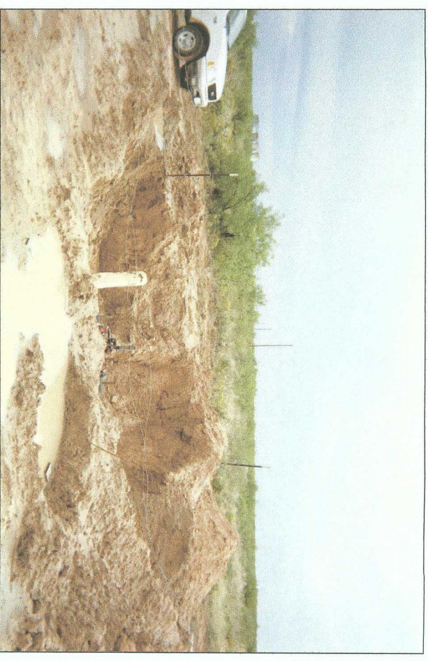
delineation trench at junction with new plumbing
