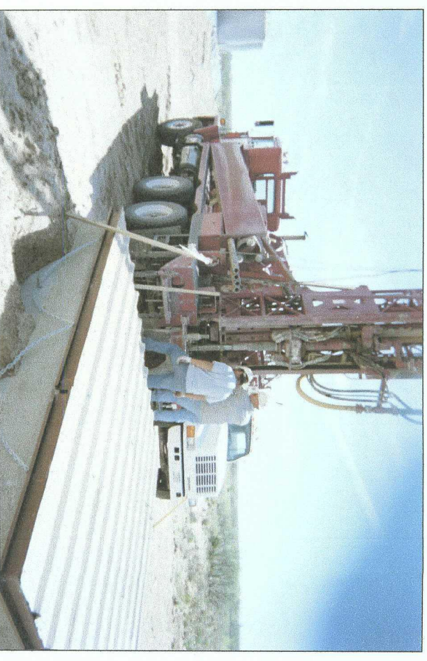
soil boring at junction box site
