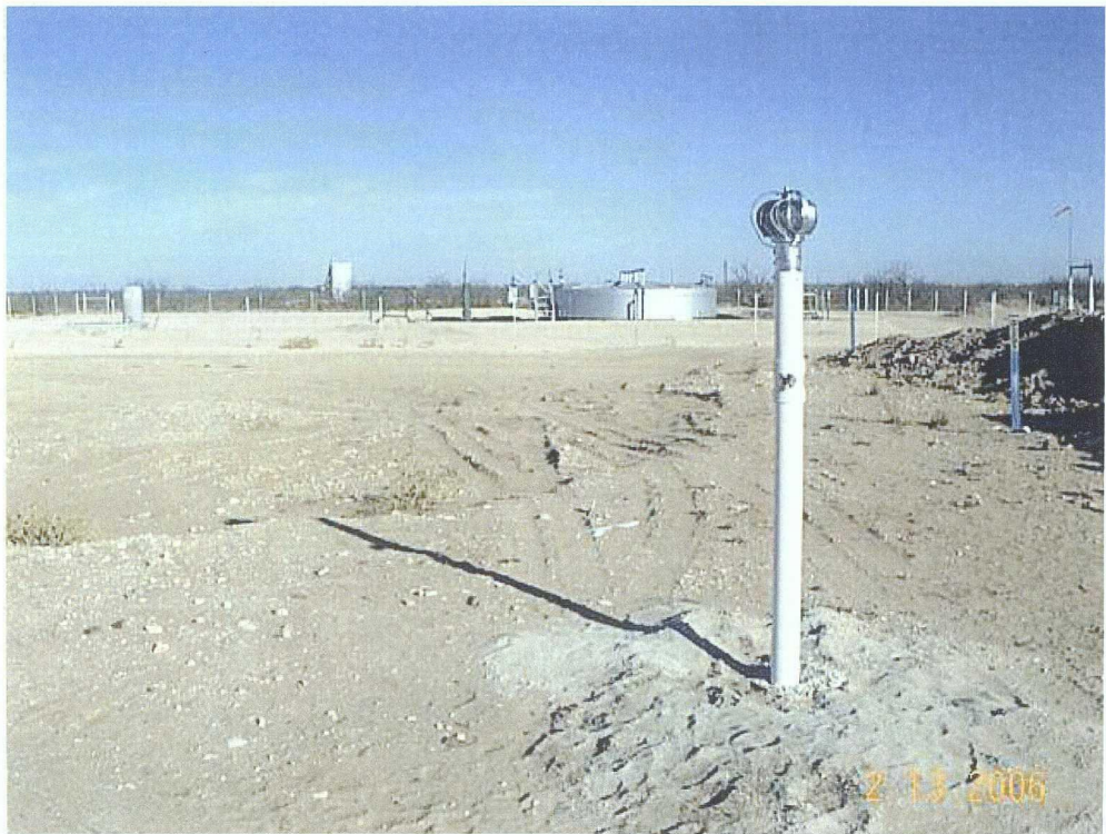
View facing east showing passive vapor extraction well at location of boring B-1.
